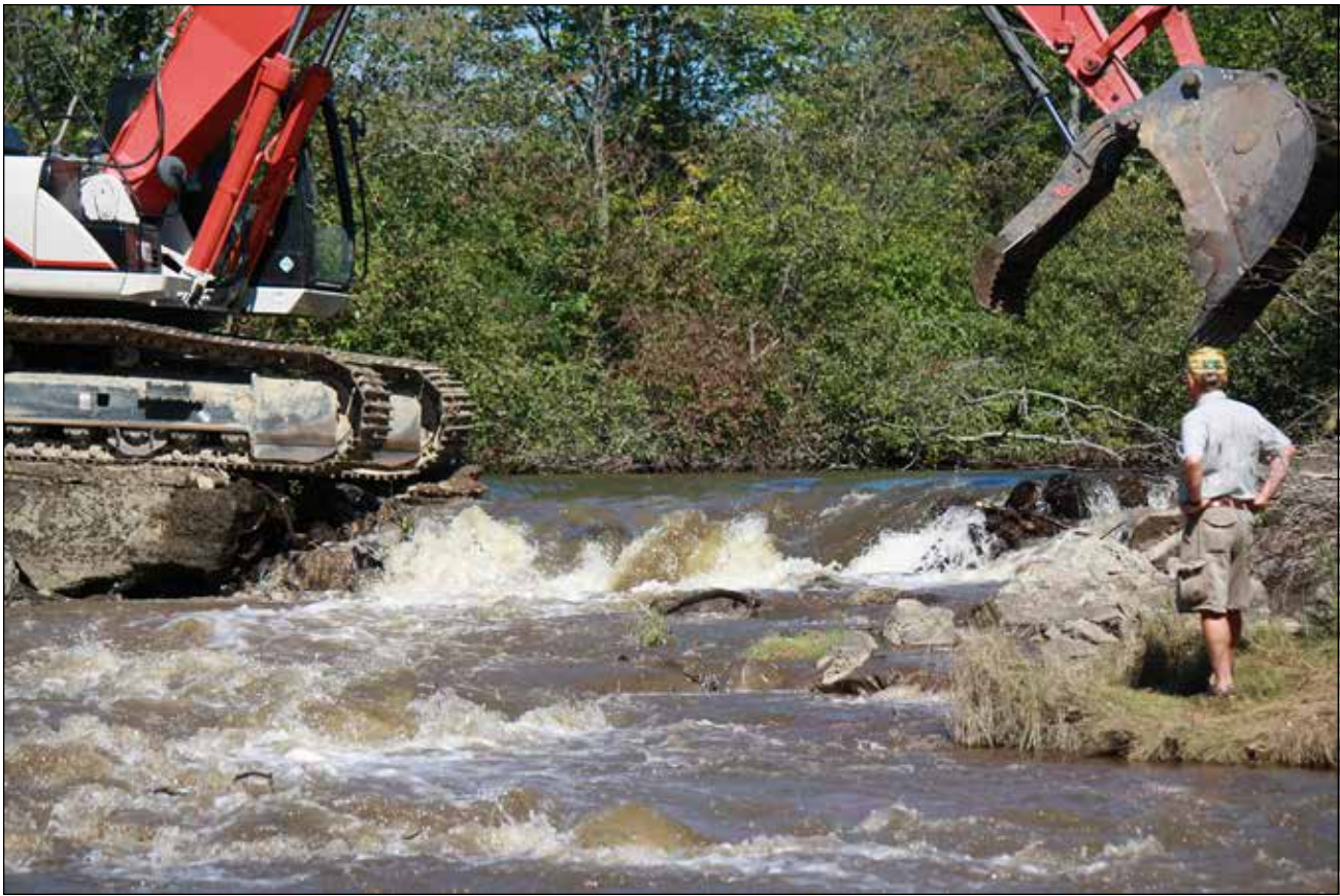
Removing a derelict dam reconnected the Kennebunk River with 7 miles of brook habitat for the first time in at least six decades.
