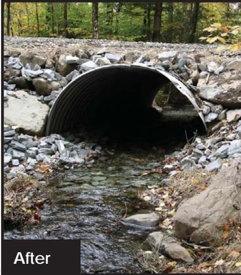
*The replacement took place on a relatively high gradient stream and will serve as a test case for the open-bottom arch under these conditions.*
